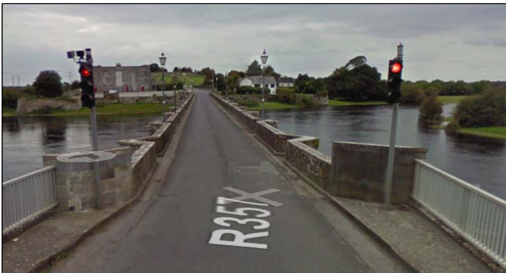
Figure 12-8: Shannonbridge bridge crossing
