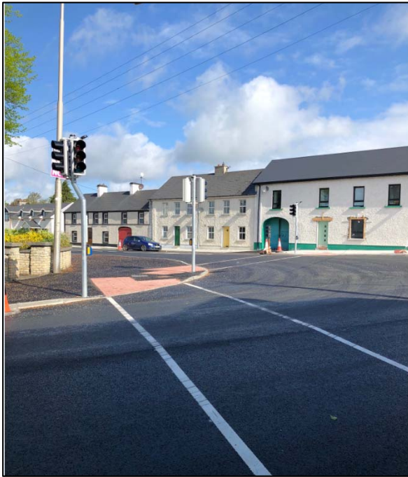
Figure 12-12: New signalised junction in Cloghan
